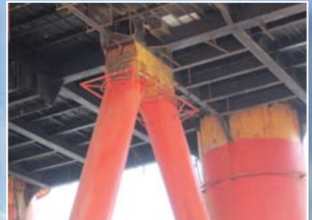
Repair Works of Helideck & Brace
