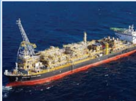
New Construction of FSO & Conversion to FPSO
