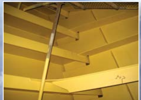
Water Ballast Tank Coatings
